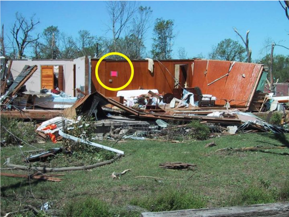
Crawford County, KS tornado 2004 Red tag placed wherever it will most likely be seen
