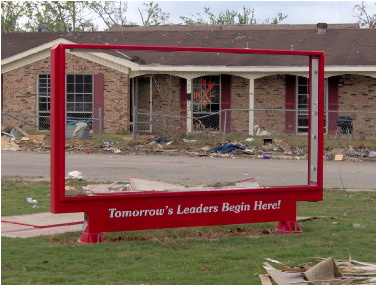
Gorenflo High School, Biloxi, MS. Hurricane Katrina's Aftermath September 2005.
